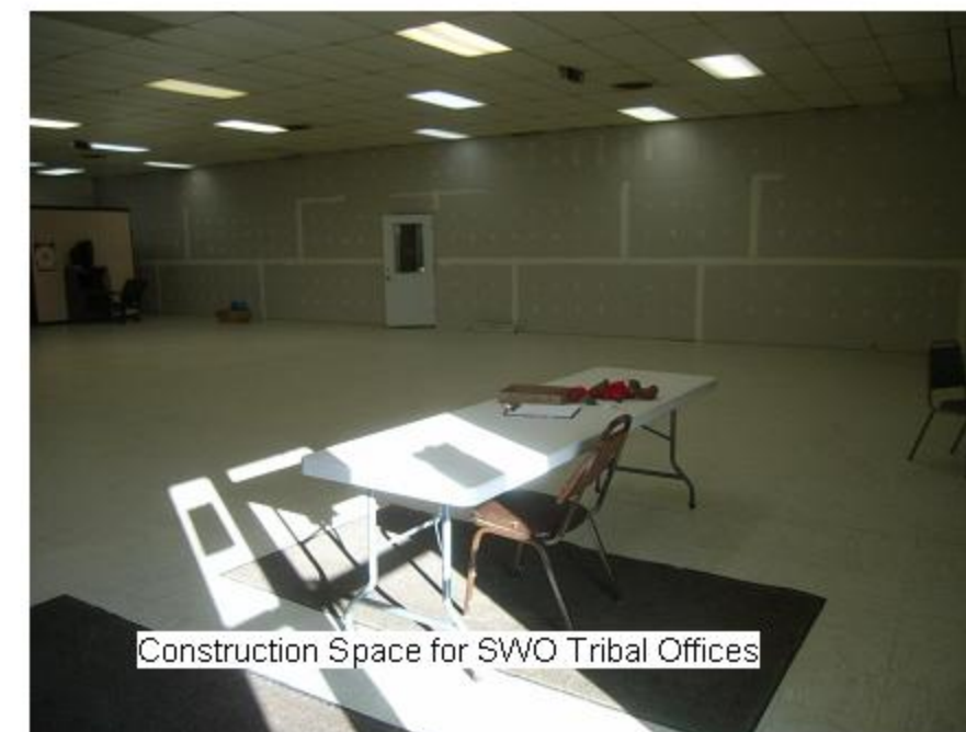
Construction Space for SWO Tribal Offices
